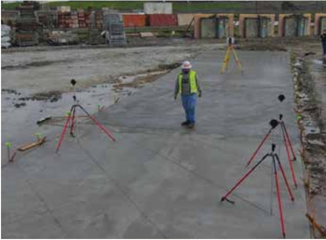
Fig. 2: A laser is used to scan the top concrete surface elevations. Previously, a laser was used to scan elevations of the compacted aggregate base substrate. Slab thickness was calculated as the difference between the two scans
